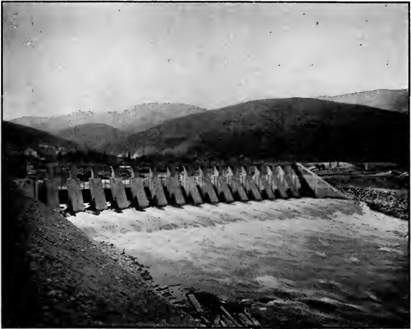
DIVERSION DAM ON TRUCKEE RIVER, TRUCKEE-CARSON PROJECT This is an "open-type" dam for discharging flood-water
